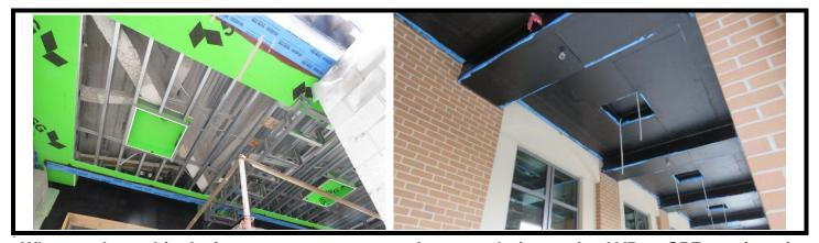
When we have this design, we must ensure we have a solution to the AVB or SPF continuation challenge, which will likely include a soffit or a secondary soffit above the architectural soffit.
