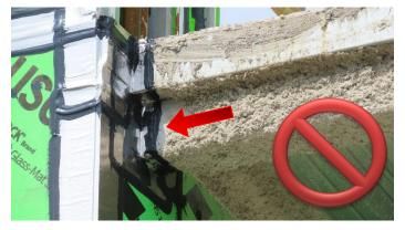
The AVB & SPF cannot be installed on or under fireproofing because it is not a proper substrate as indicated by AVB manufacturers, and has not been fire tested to be on top, and cannot achieve the adequate pull-off strength.
